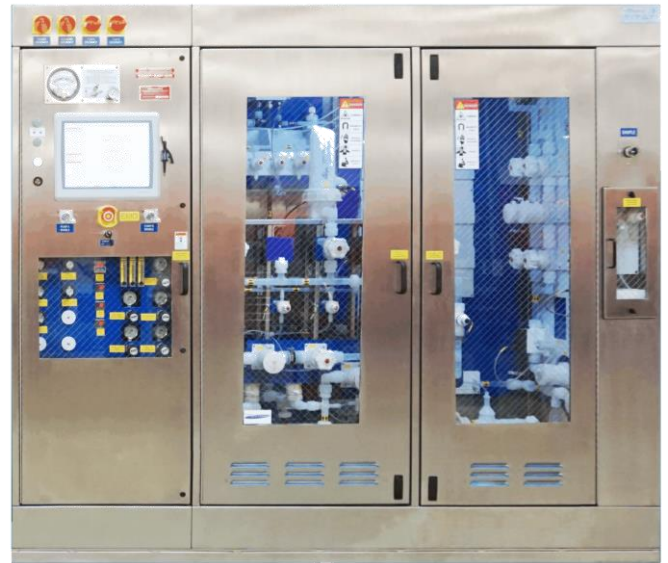
Control Cabinet and Solvent CDU
