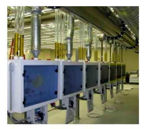
This turnkey piping system installation is a quality example of the onsite services performed by **DFS**. We were contracted to design, install and commission the bulk chemical distribution system piping for a Solar Cell Manufacturing Facility. This system is all double-jacketed piping for Sulphuric Acid, Sodium Hypochlorite, Sodium Hydroxide, Sodium Sulphite & Sodium Chloride.
