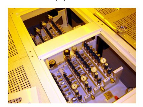
At **Diversified Fluid Solutions**, we are experts at all types of process tool and equipment installation. Shown here is an example of our patented (Patent # 7.039.999 B2), raised access floor (RAF), drop-in gas module for a semiconductor cleanroom. We can provide hook-up needs or requirements for all utilities - electrical, mechanical, process gas, water, chemical, controls, etc.
